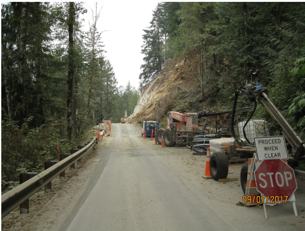
Above: Slope excavation work area.
