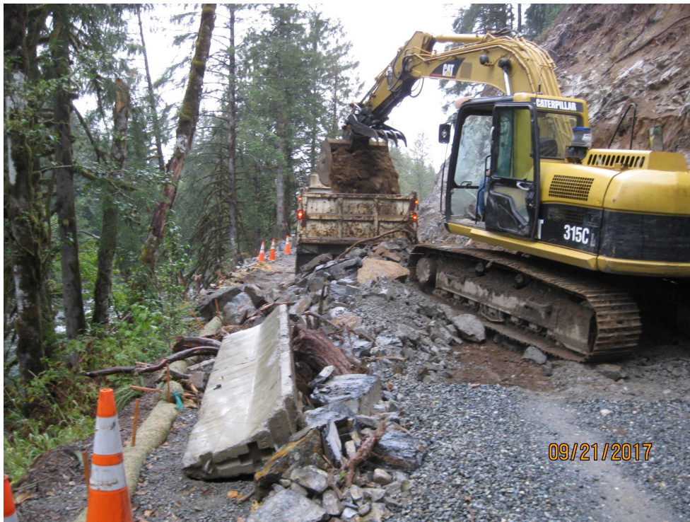
Above: Loading and hauling the slope excavation.
