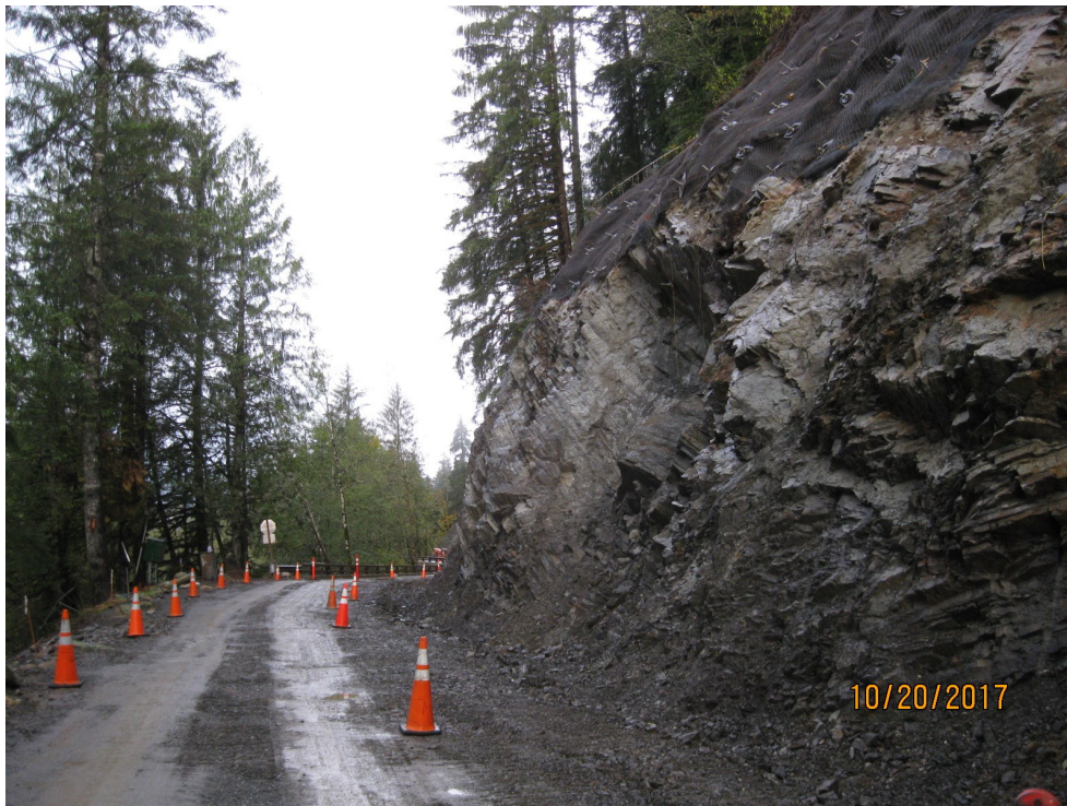
Above: Widened roadway.
