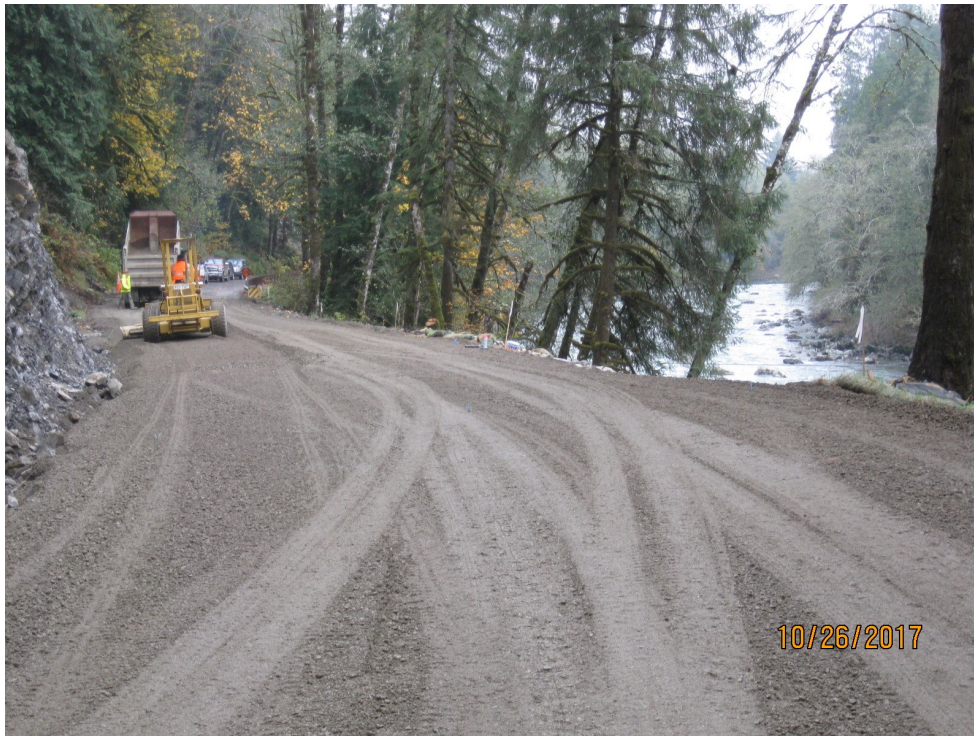
Above: Grading roadway surfacing rock.
