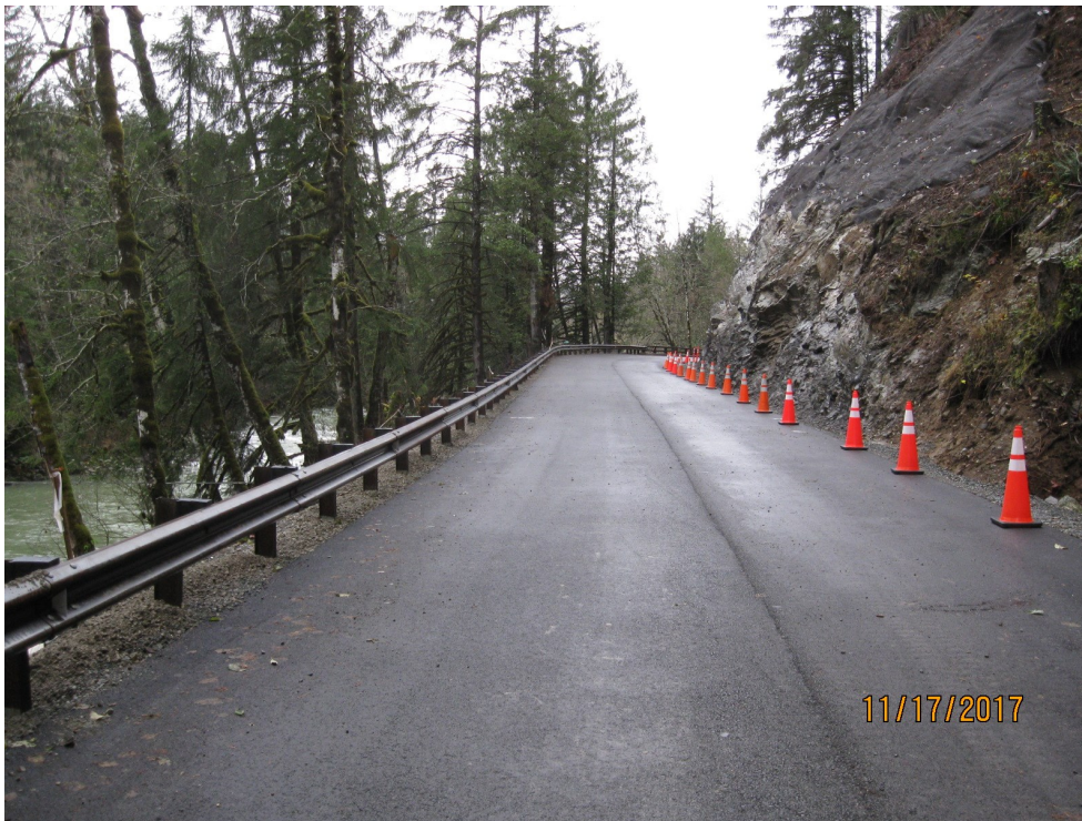
Above: Completed roadway with new guardrail.
