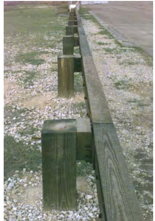
Type A steel-backed timber guardrail
